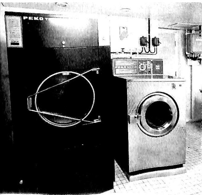
Washing Room equipped with Wärtsilä Washing Machines
