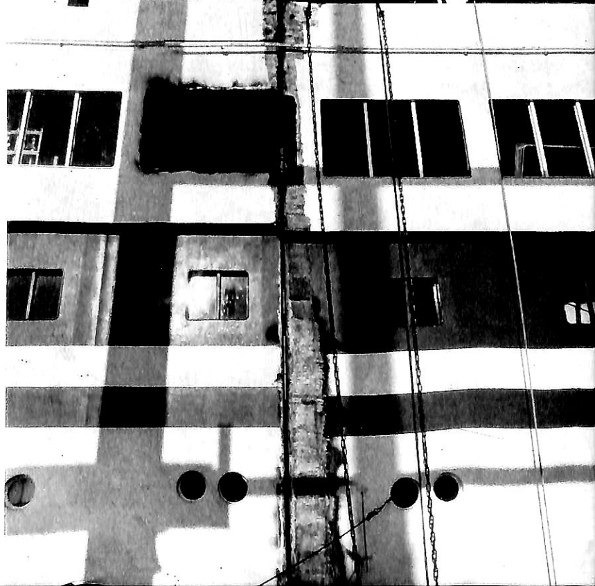
Cutting operation in progress
