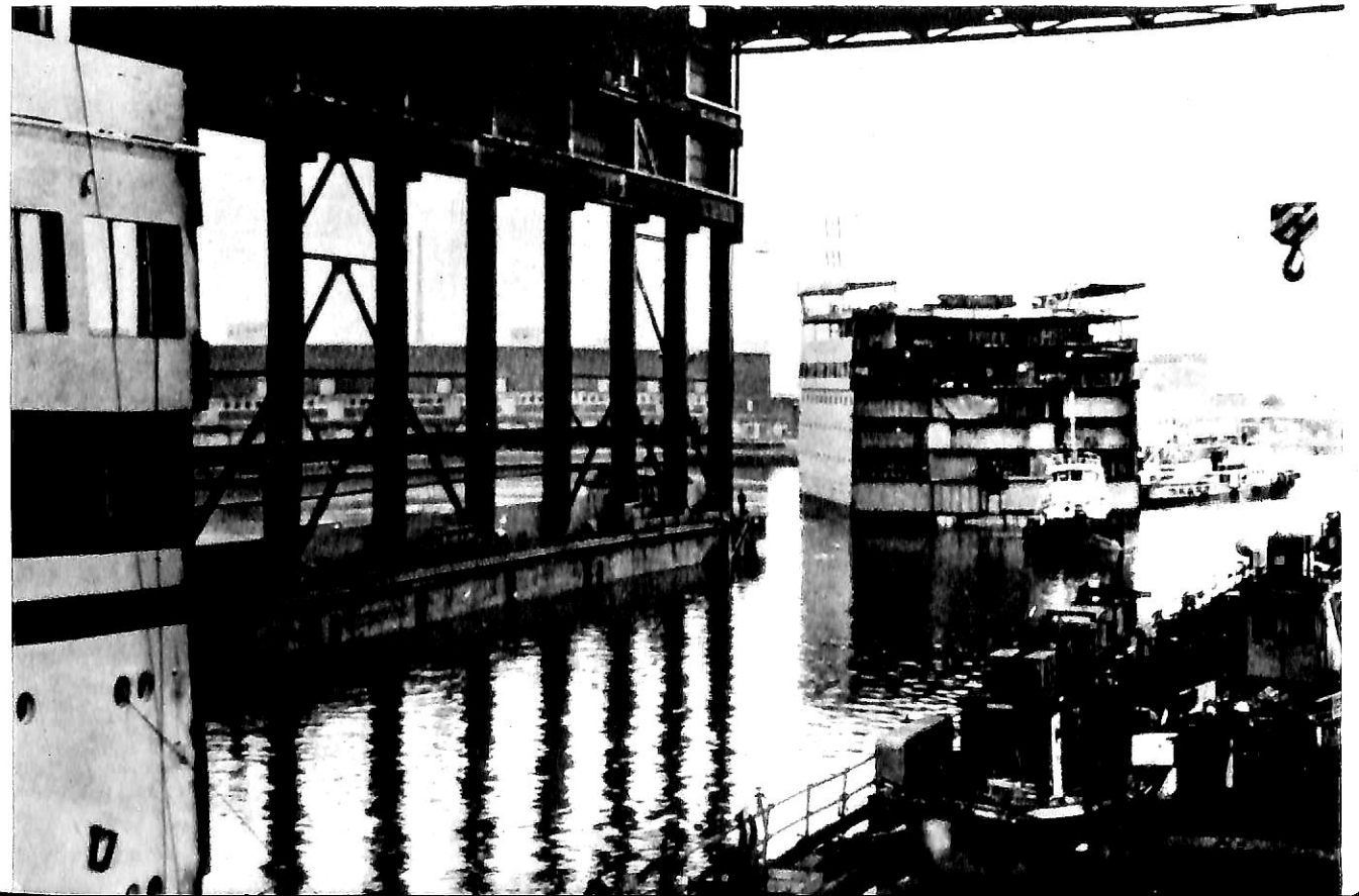
The midsection is being brought into the building
