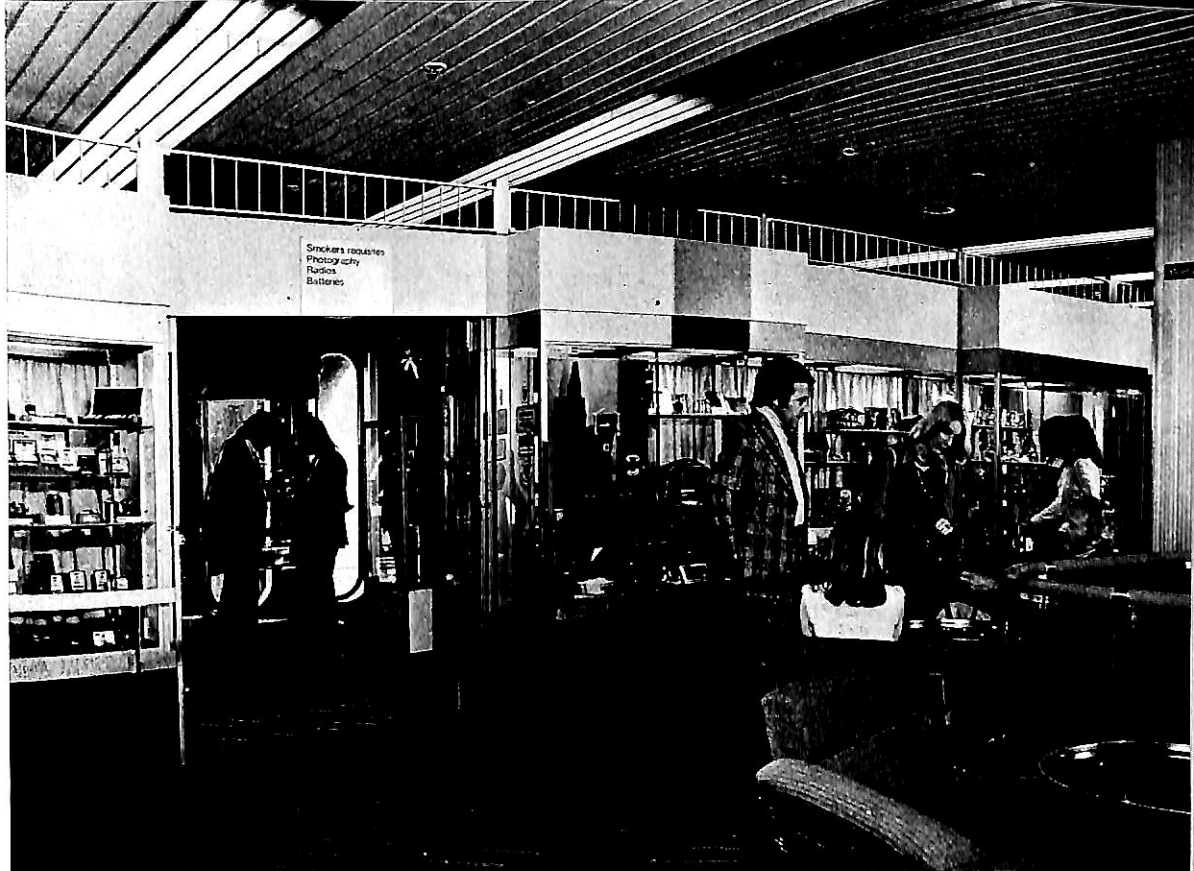
The reconstructed Shopping Arcade at Boat Deck level. Photographed in January 1974.
