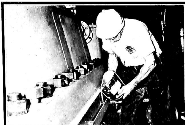
CHOCKFAST ORANGE 610TCfの注入作業
