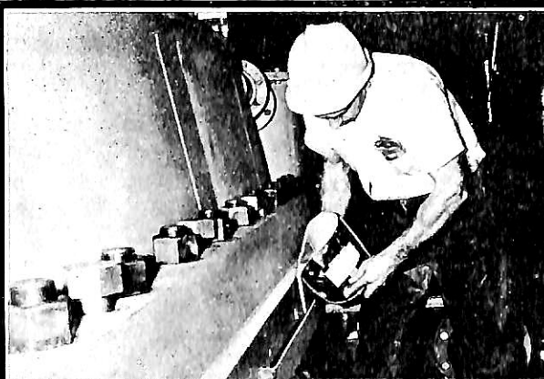
CHOCKFAST ORANGE 610TCfの注入作業
