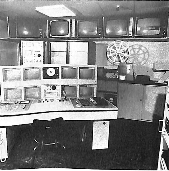
TV control room
