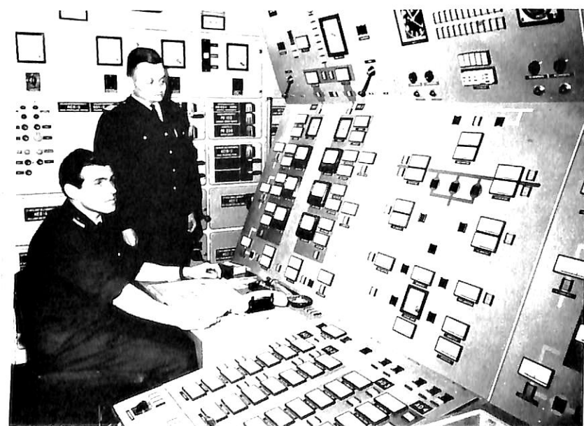
Engine Control Room
