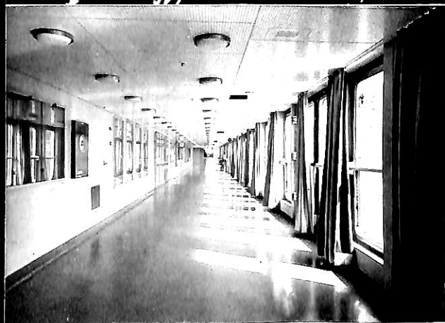
← 1st class covered promenade deck
