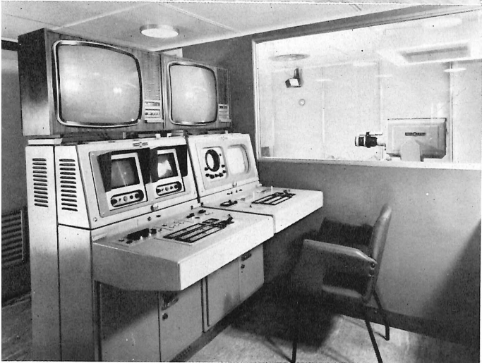
TV control room (R.)
