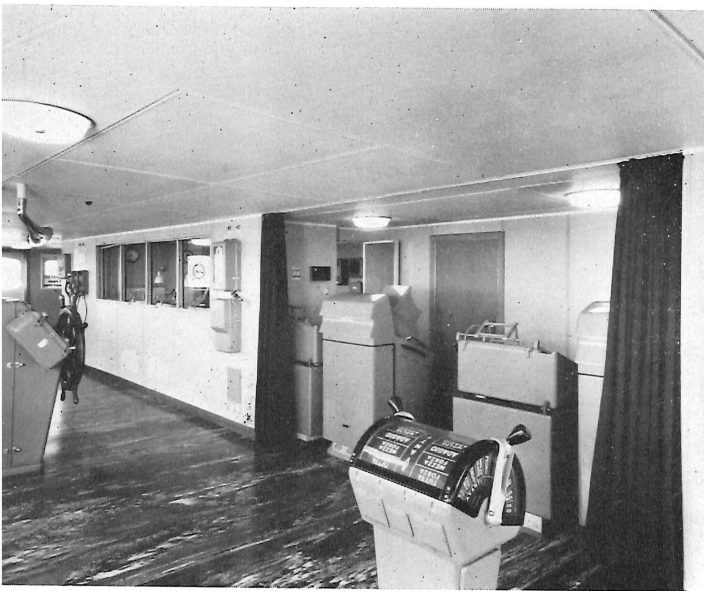
Wheelhouse looking aft (Raffaello)
