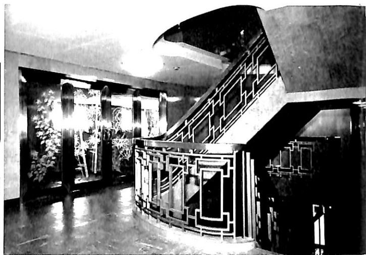
Hall on bridge deck
